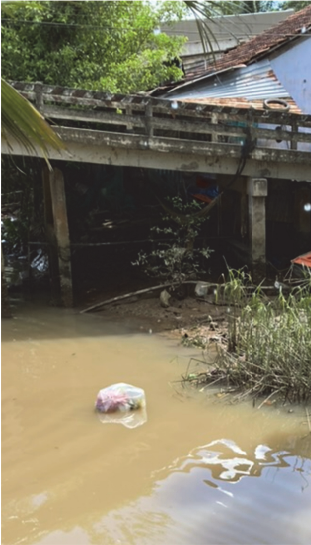
Figure 6: Rural Area in the Mekong Delta: Waste from a Local is Regularly Thrown from the Bridge into the Water
